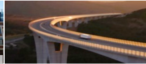
KRINKAL BRIDGE - SLOVENIA
